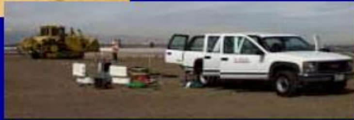
SASW Data Acquisition
